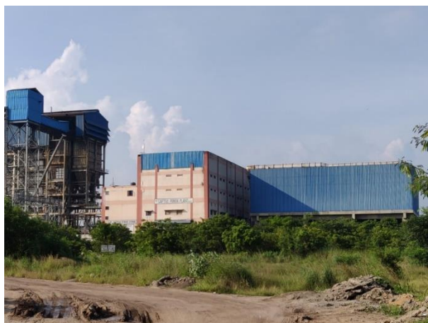
Captive Power Plant - II
